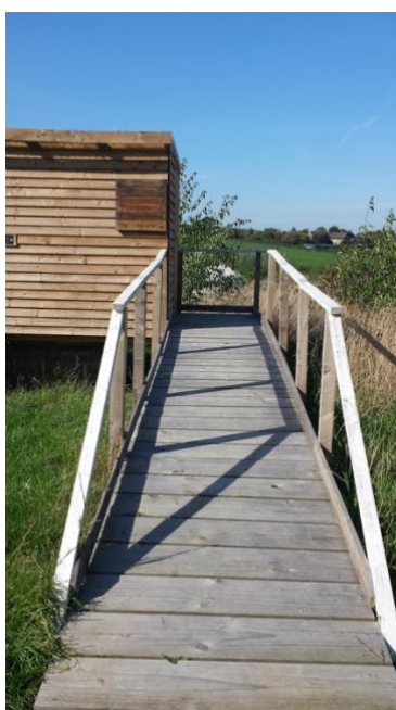
Wheelchair accessible Tree Bog at Whistlewood Common – photos by Anne Bramley (note – suitable uprights are still to be added to the handrails of the ramp)
